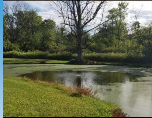
A stormwater pond with excessive vegetation due to the lack of a vegetative buffer
