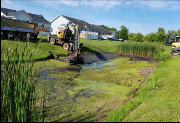
A stormwater pond is excavated and depths are re-established due to excessive vegetative
