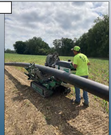
Fusing and installation of the pipe in August 2022
